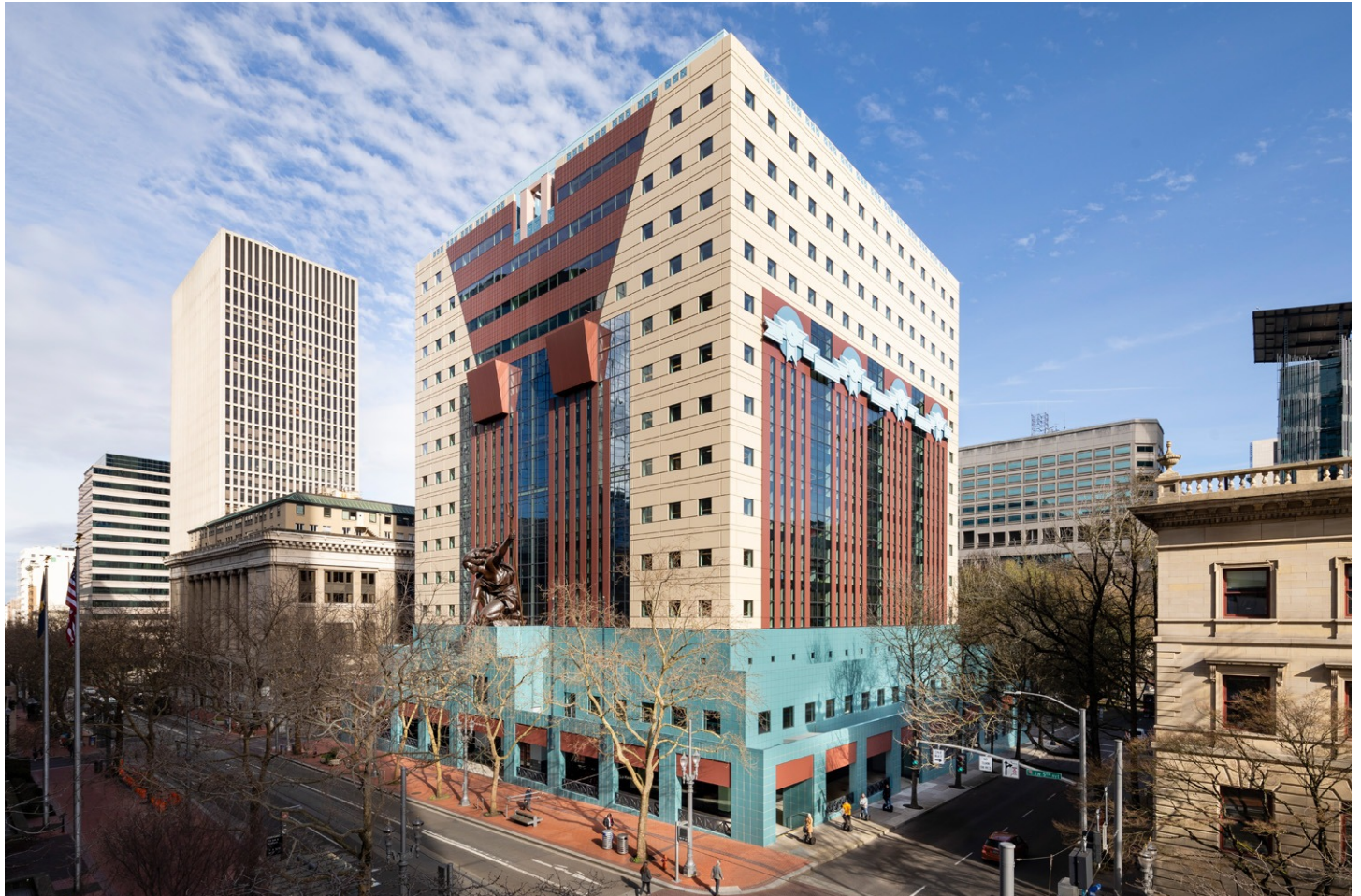
The Portland Building Reconstruction
