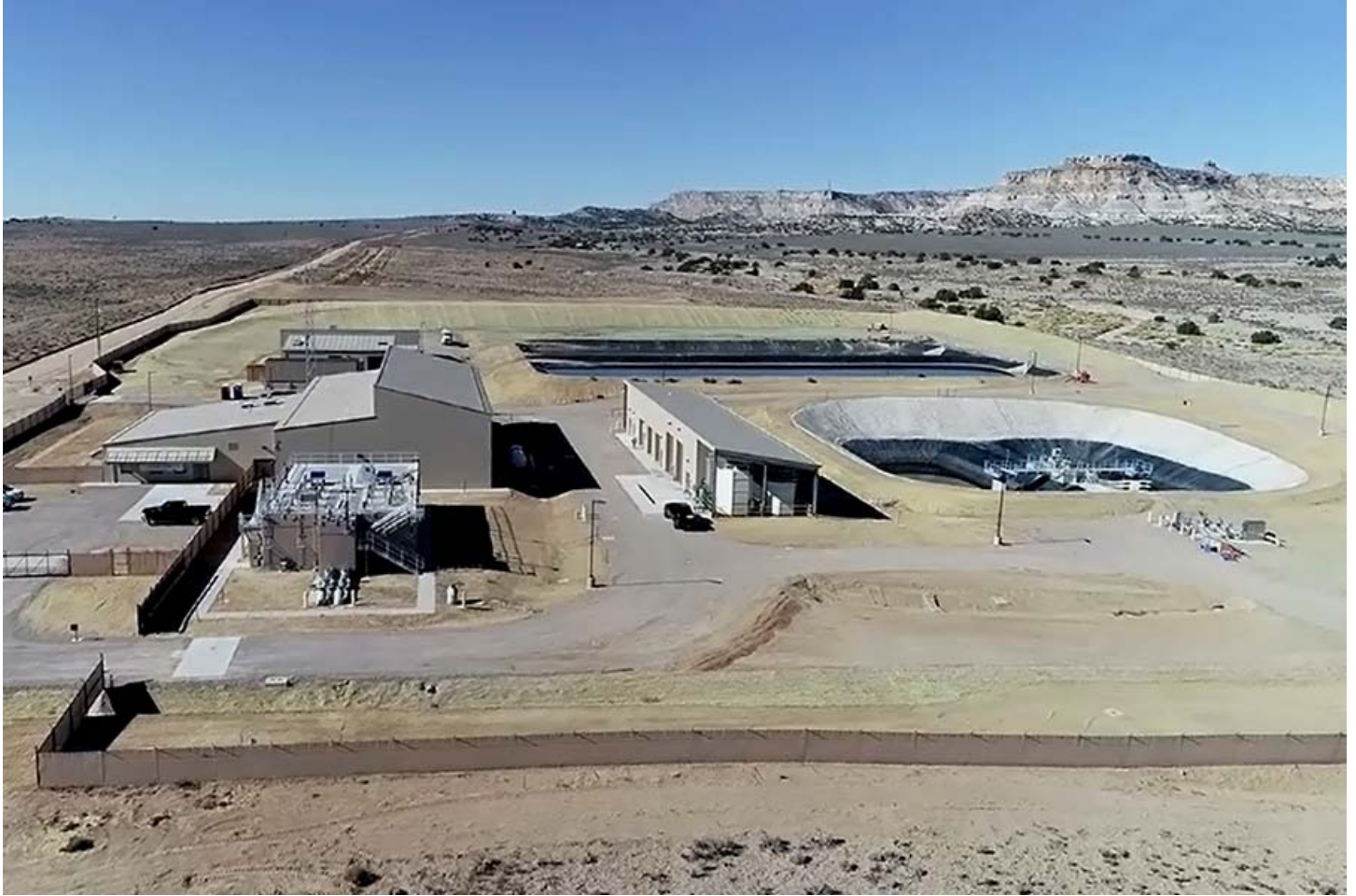
Cutter Lateral Reach 21 Water Treatment Plant and Associated Items, Navajo Gallup Bloomfield, New Mexico
